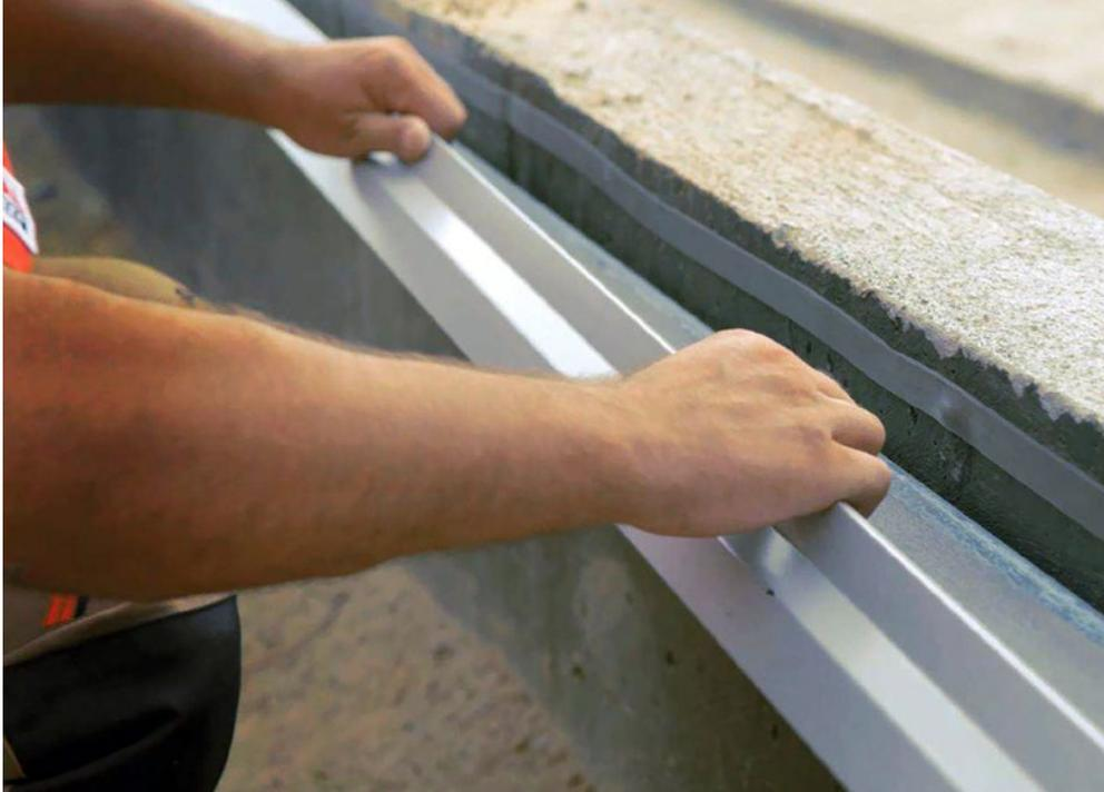
It should be remembered that the casing made of BALEX METAL sandwich panels is not a system and the assembly method shown above is only an example. More plinth detail solutions can be found in the technical catalogs available on the website.
