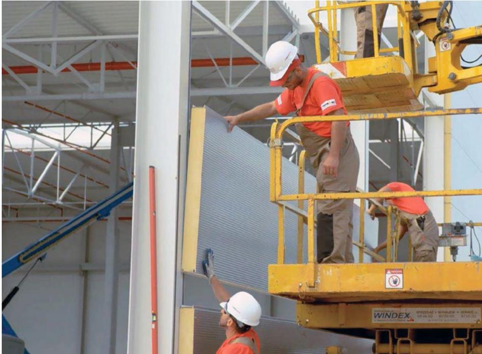
Subsequent panels should be pressed so that no gaps remain in the lock.
