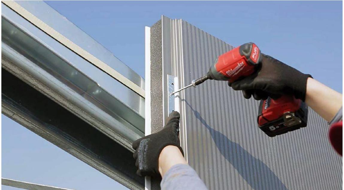
Remember to choose the right fasteners - more information in section 4.1.6. When installing panels with hidden fastening, it is recommended to use stress redistributors (as in the picture above).
