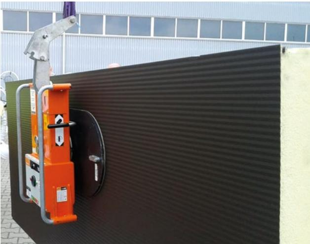
*Selection of a vacuum lifter depends on the dimensions of the sandwich panels and the core material. That's why selection of number, spacing and type of suction cups need to be done for every case separately. Vacuum lifter rental companies offer such selection in standard. Such help is recommended because improperly selected equipment can (in extreme cases) lead to delamination of the panel cladding from the core.*
