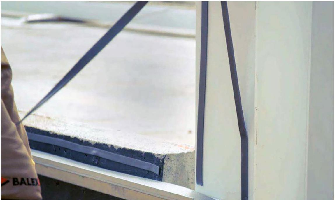
In the case of a wide support, remember that stick the tapes as close to the edge as possible.
