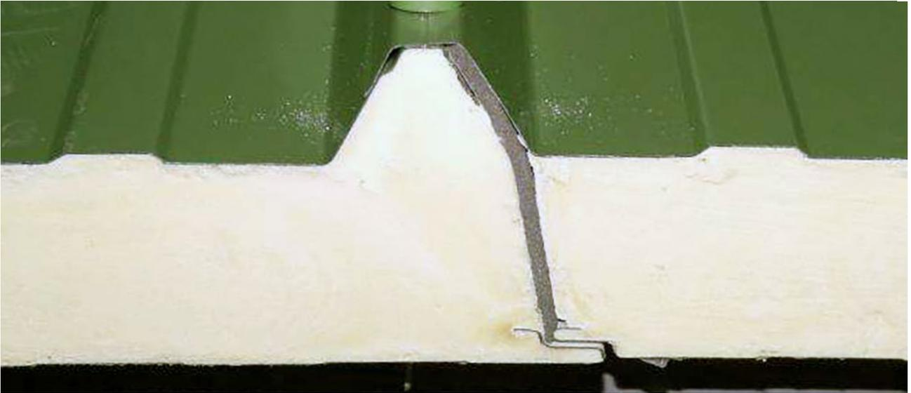
Correctly pressed BALEX METAL panel lock
