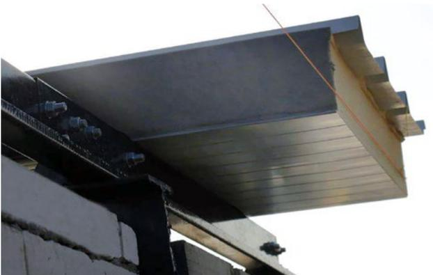
It is important to lay the panel precisely. A construction cord can be used for this purpose.
