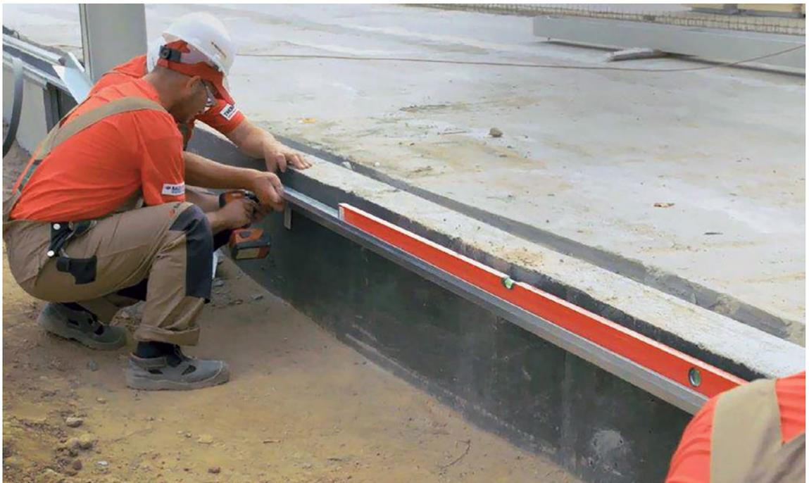
During assembly, it is necessary to constantly check the level of the profile with a long spirit level.
